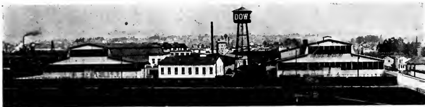
A general view of the Dow plant. These shops form one of the most complete engine works on the Pacific Coast.
